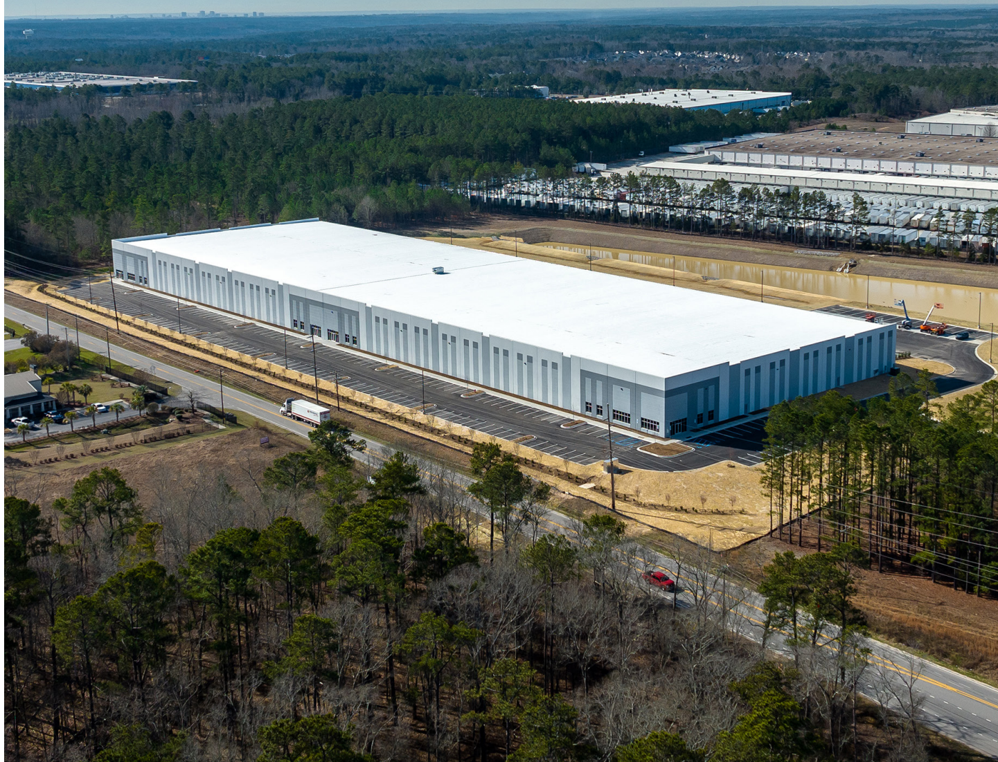
Above: Carolina Pine Industrial Park, Columbia, SC
